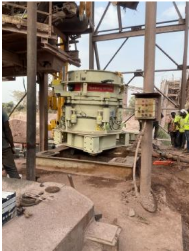
Photographs of the new tertiary crusher and the new screening unit being installed
