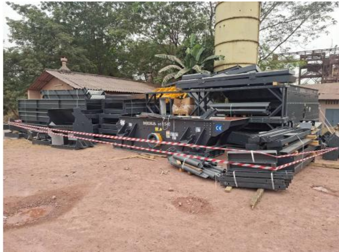
Photographs of the new tertiary crusher and the new screening unit being installed
