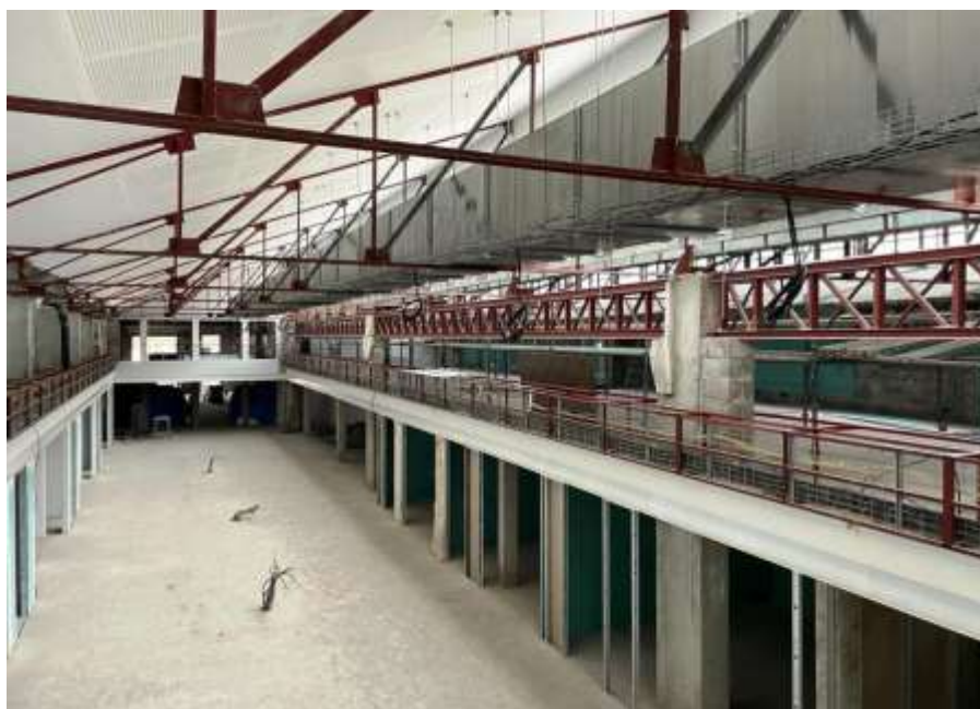
Chantier Silikin Village Phase III
