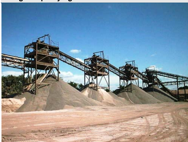
Carrigrès' quarrying site
