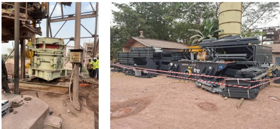
Photographs of the new tertiary crusher and the new screening unit being installed
