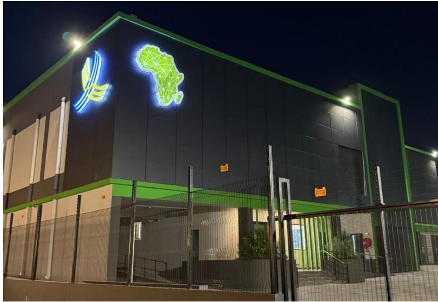
Data centre OADC Texaf Digital
