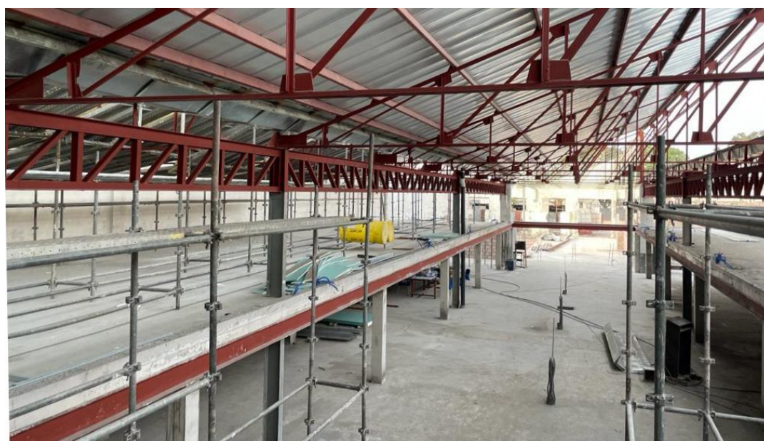
Chantier Silikin Village Phase III
