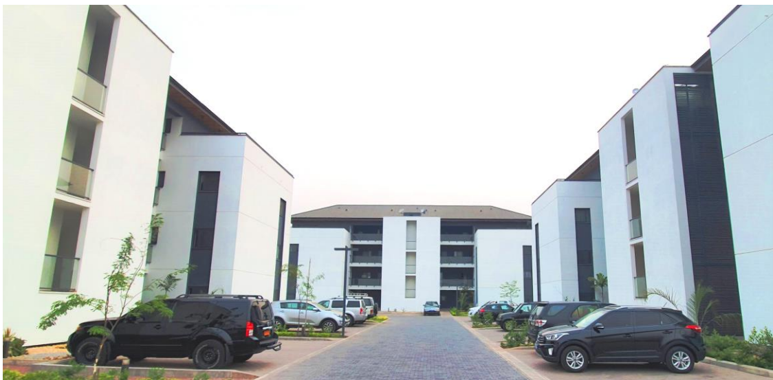
Bois Nobles courtyard
